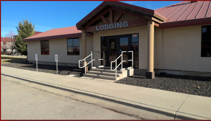
Bldg. 00710 West End
