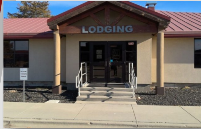
Construct ADA Access
