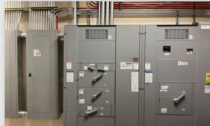
Repair Electrical Loads
