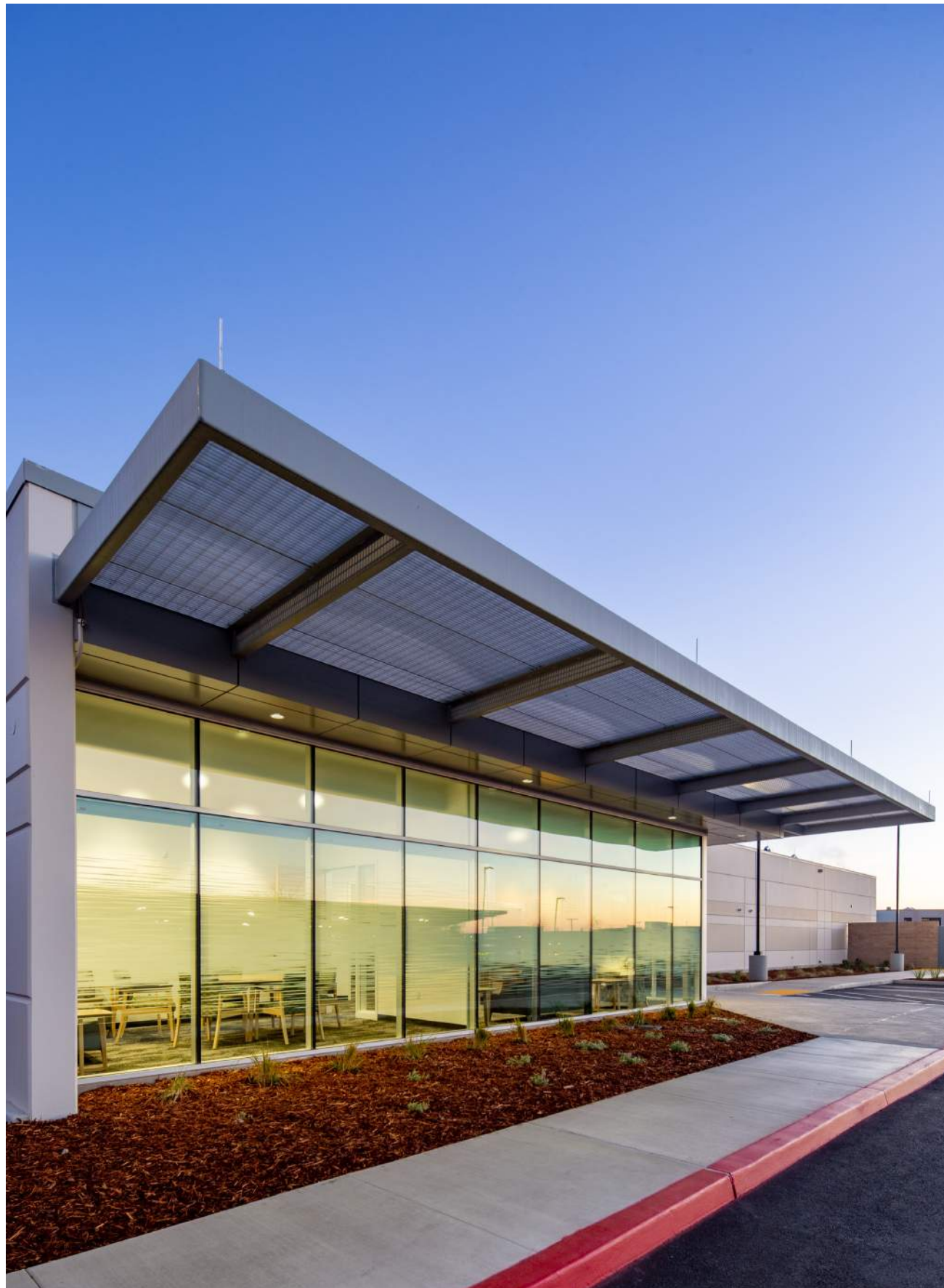
Placer County Coroner Facility
