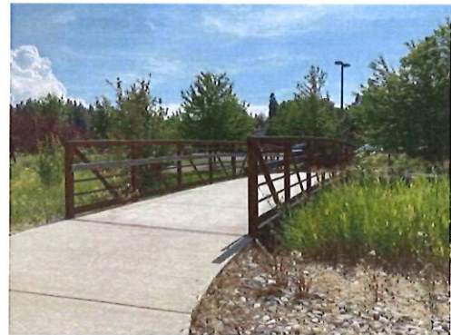
Existing Prefabricated Pedestrian Bridges spanning Paradise Creek.
