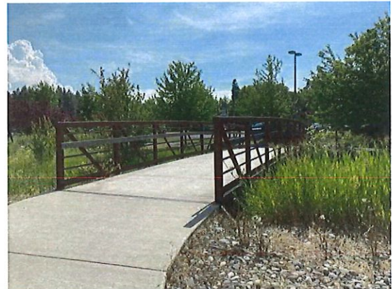
Existing Prefabricated Pedestrian Bridges spanning Paradise Creek.
