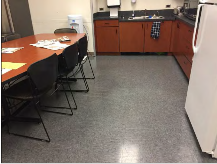
13. View of the new non-asbestos grey sheet vinyl floor tile found in several locations throughout LBJ Building.
