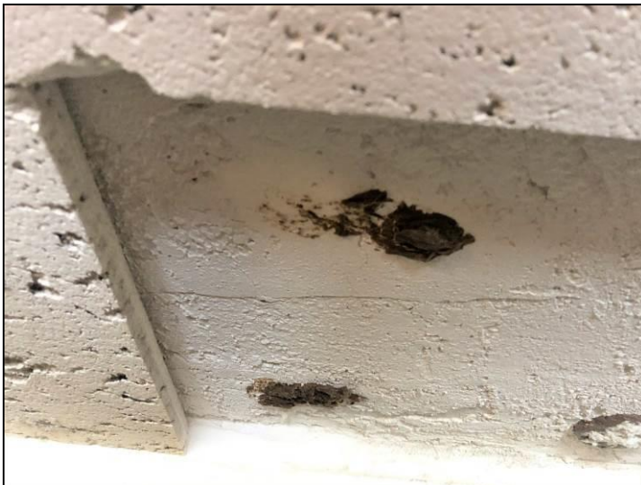
9. View of the non-asbestos 12"x12" concealed spline ceiling tiles and the non-asbestos fiberglass duct insulation found in various locations throughout the building.
