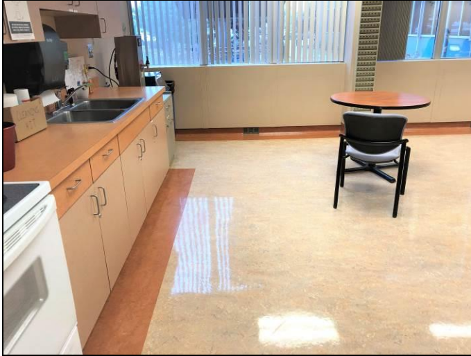
16. View of the new non-asbestos sheet vinyl flooring and cove base found in the large breakroom located on the first floor.
