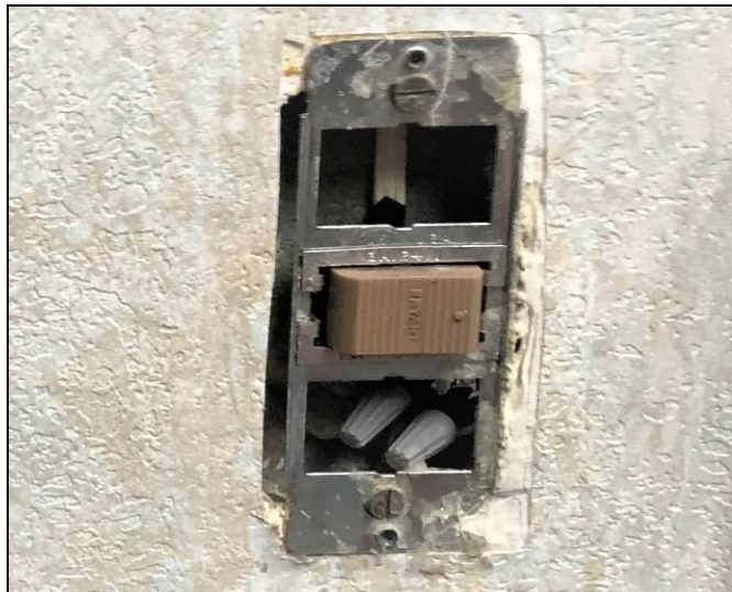
11. Closeup view of the non-asbestos vinyl wall covering found in various locations within the main building.
