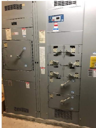
The Existing Main Switchboard
