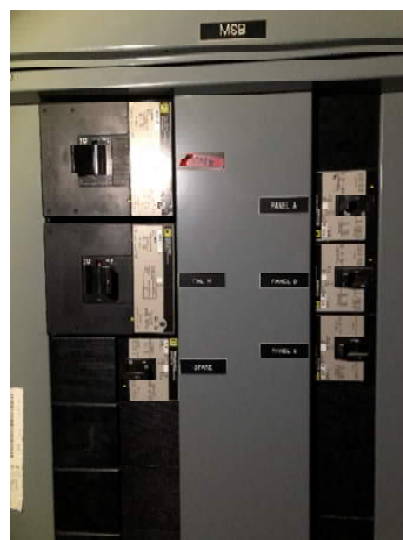
MSB LOAD BREAKERS
