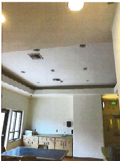
Existing Dayroom Ceiling
