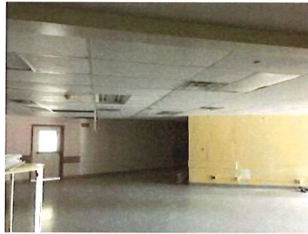
MAIN LOBBY CEILING
