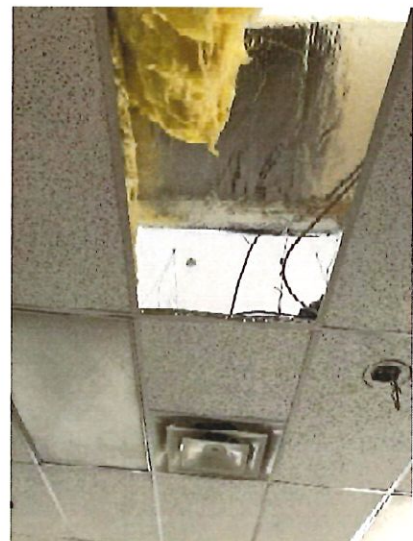
DAY ROOM CEILING SHOWING DAYLIT AREA ABOVE DROP CEILING
